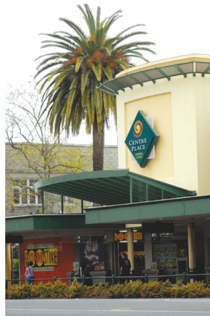
Centreplace Mall, Ward and Victoria Streets, Hamilton
