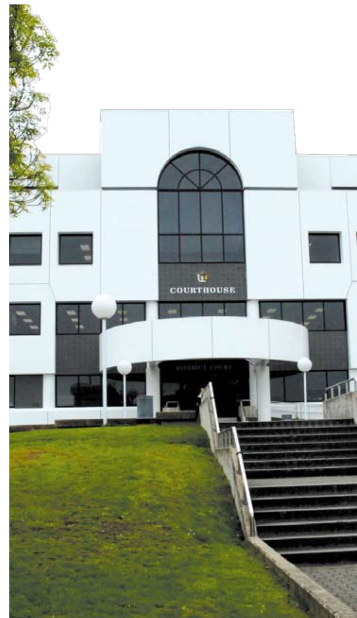
Hamilton Courthouse, Cnr Anglesea and Bridge Streets, Hamilton
